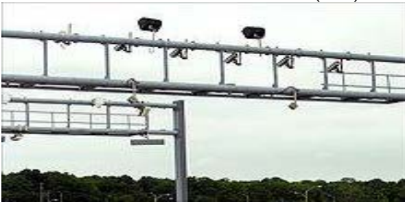
Figure 1. Ontario's road 407- use of automatic range plate recognition
